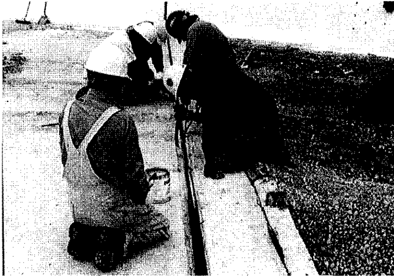
Figure B.18 Installation requires working in small increments
