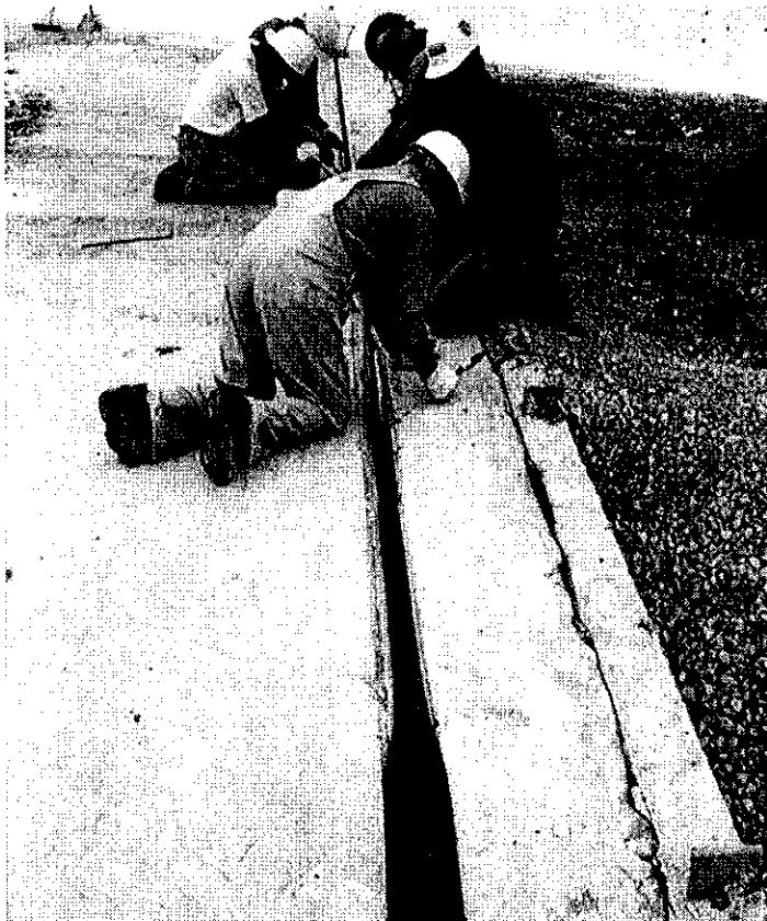
Figure B.16 Seal is installed in one piece from end to end
